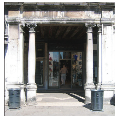
F3 Renovation of Clock tower in Piazza San Marco
